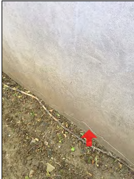
16. Parging damaged or missing
