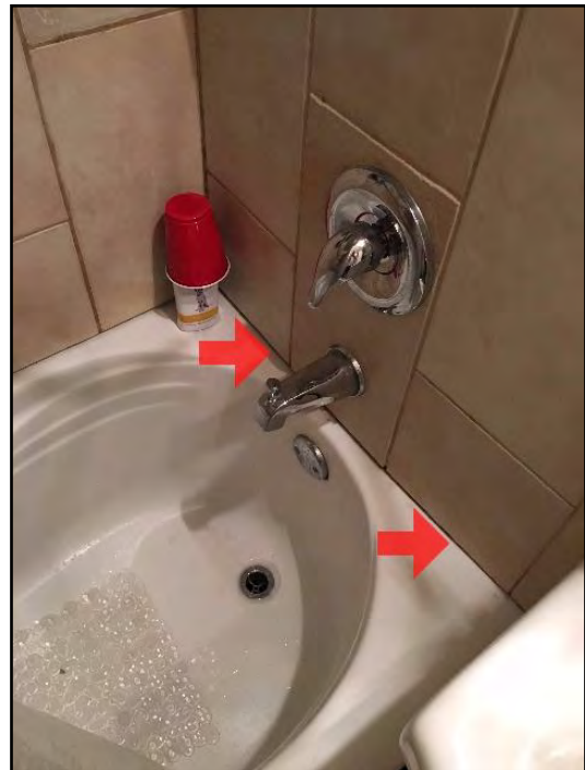
42. Caulking loose, missing or deteriorated
