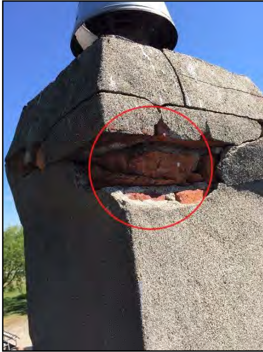
26. Loose, missing or deteriorated masonry
