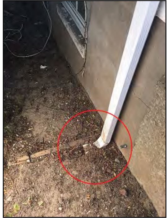
4. Downspouts end too close to building
