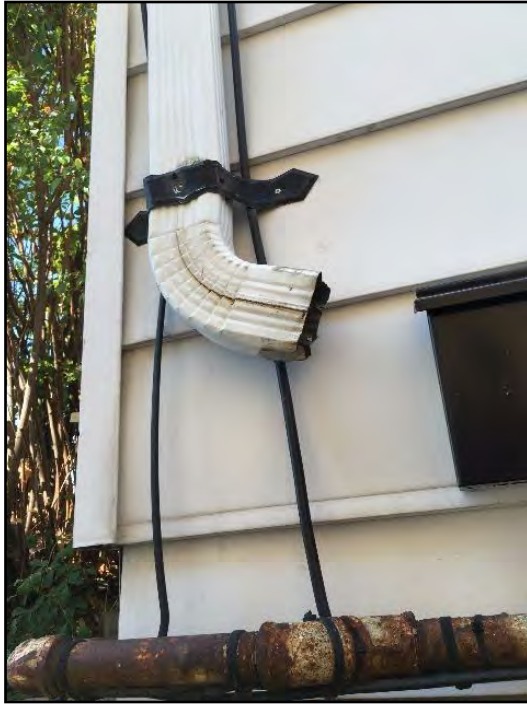
3. Downspouts end too close to building
