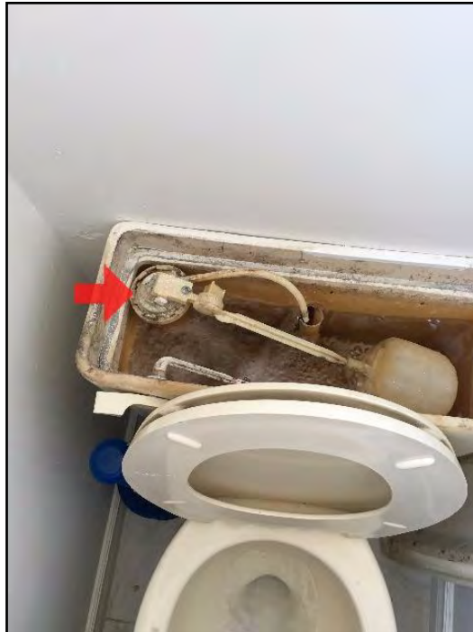
40. Replace valve in toilet as it is not...
