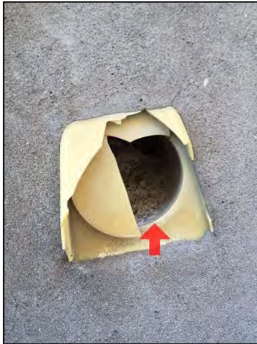
1. Damaged or Dirty Vent Cap
