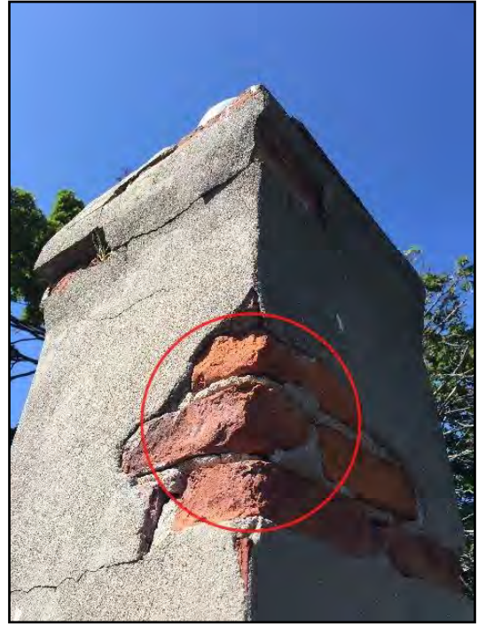
27. Loose, missing or deteriorated masonry
